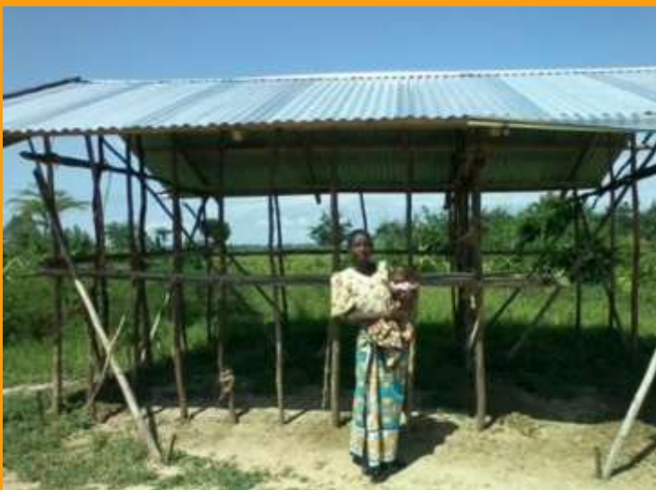
Renovation work in progress
